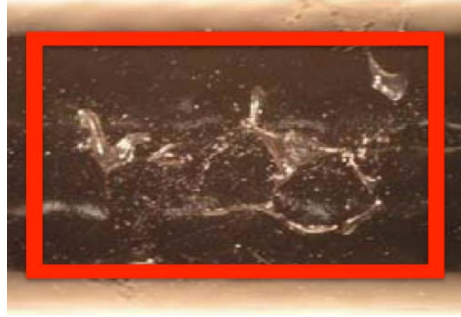
Peeling of the universal cord tube coating
