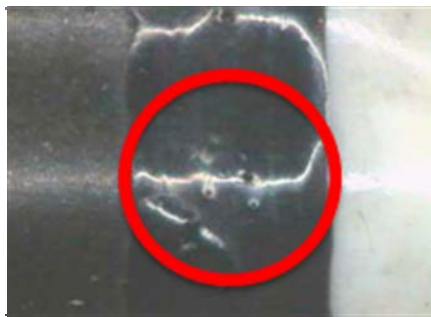
Bubbling of adhesive at bending section cover
