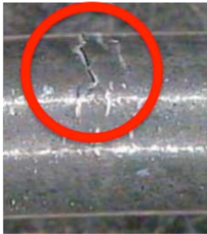
Cracking of the insertion tube
