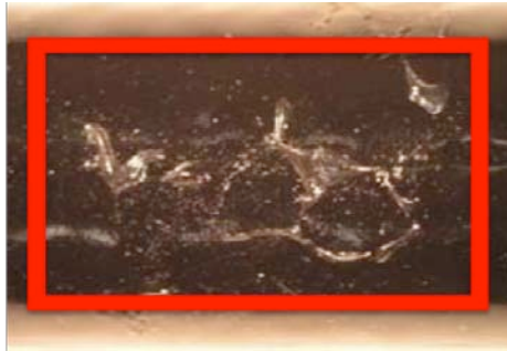
Peeling of the universal cord tube coating
